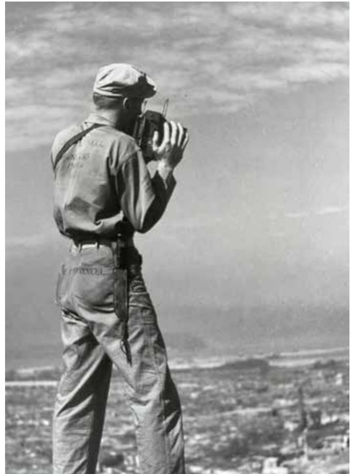
Figure 4b. Standing on the Roof
