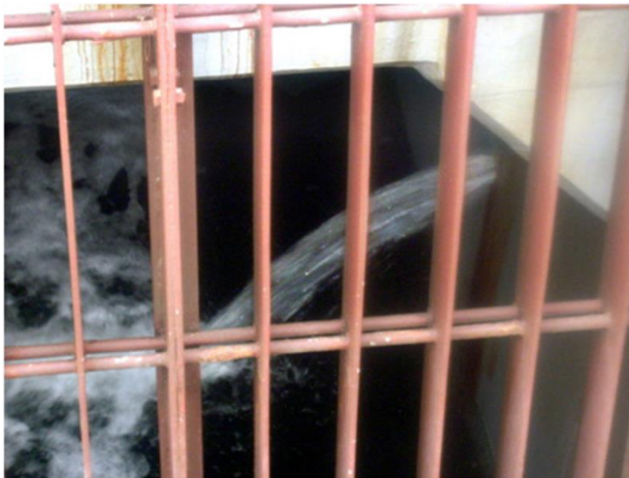
Radioactive water leaks into the sea April 2 from a crack in a pit wall near the water intake of the No. 2 reactor at the Fukushima No. 1 nuclear power plant. (TEPCO)
