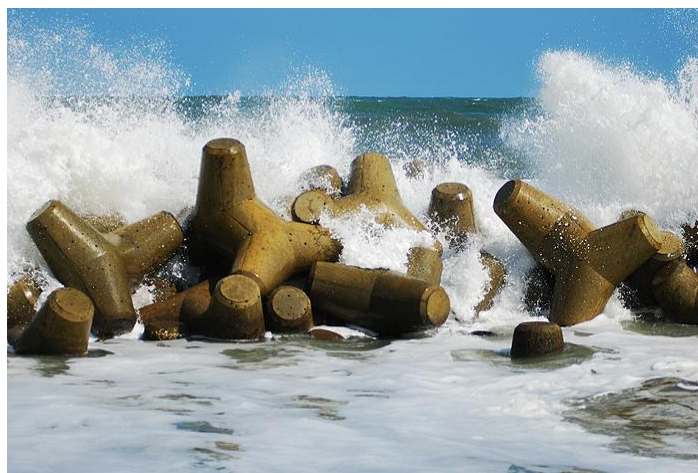
Concrete "tetrapods" on the Fukushima coast, used to minimise erosion (Mike Beddall photograph)
