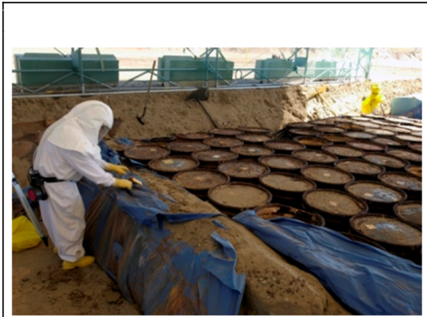
Worker with radioactive waste at Hanford
