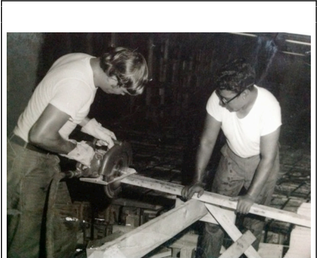
U.S. service members work beneath decks ensuring the chemical weapons fit snugly together. Tim Gravelly
