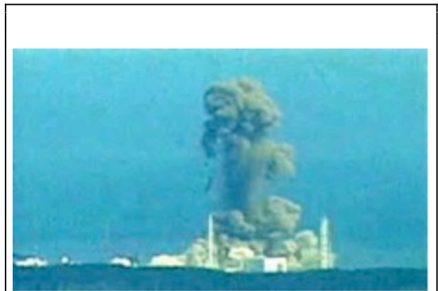
Explosion at Fukushima Daiichi Nuclear Power Plant March 2011
