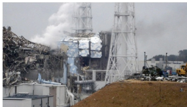
Damaged reactors at Fukushima Daiichi
