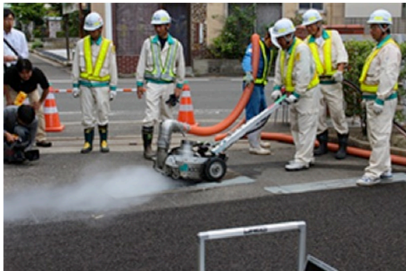
Decontamination work at Fukushima University
