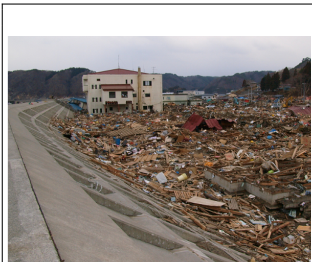
Figure 4. Tarō in the wake of the March 11, 2011 disaster. The great seawall was not tall enough to hold back the tsunami. Source (accessed 5-13-2011)
