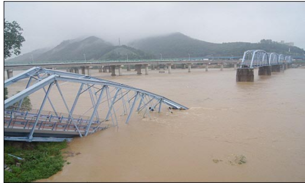
Collapsed Waegwan Railroad Bridge, from Ohmynews June 26, 2011 28
