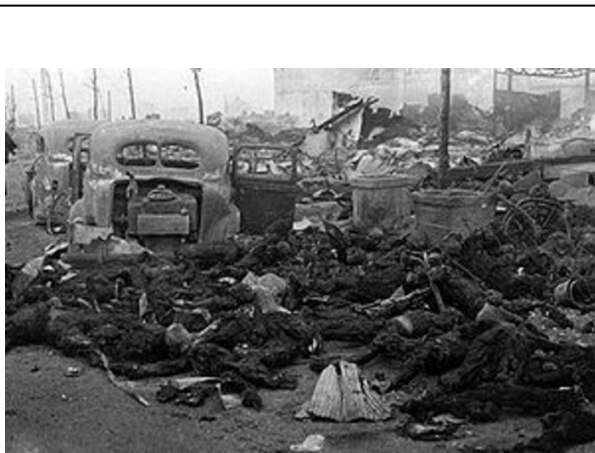
Charred remains in Tokyo March 10, 1945.
