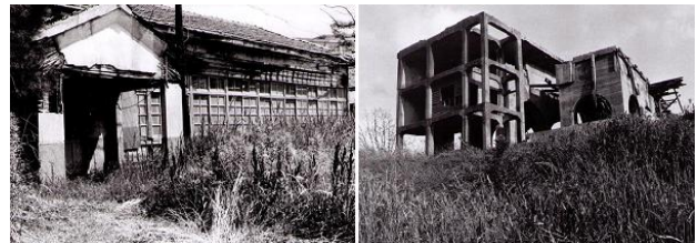
The abandoned Aso Yoshikuma work office (left) and ruined Aso Yoshikuma mine buildings in the late 1970s. Neither structure remains today. (Hayashi Eidai photos)
