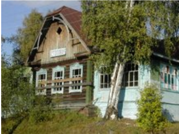
The closed dining hall of a former state-owned tourist base in Artybash.
