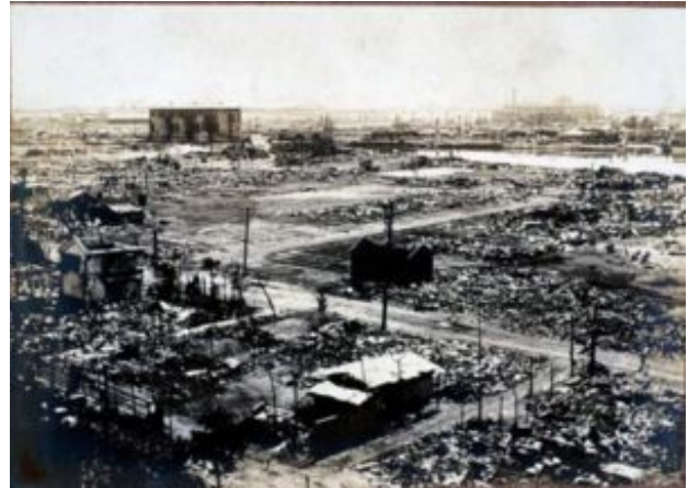
Earthquake destruction in Yokohama
