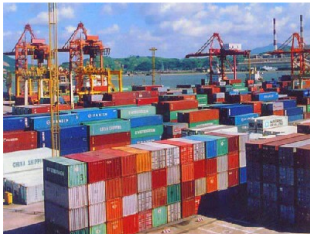
Containers at Fuzhou port
