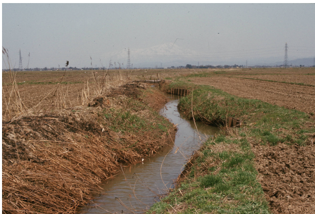
An old unlined branch canal
