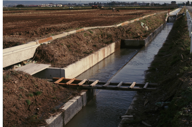
The same canal after construction, late 1970s
