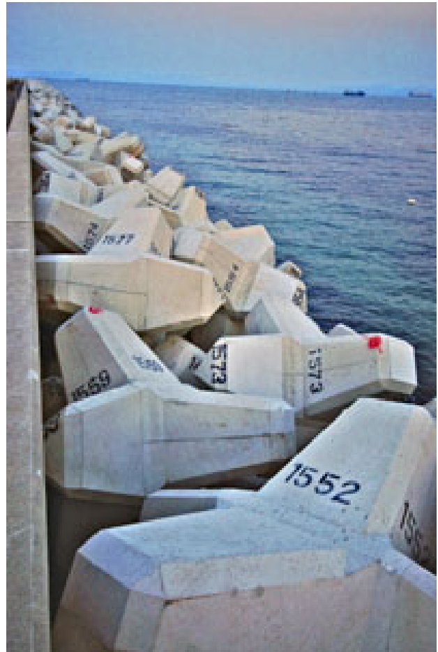
Tetrapods lining the coast at Yokosuka. Photo by Aoyama Ken
