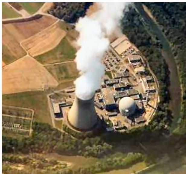
Nuclear power station at Leibstadt, Switzerland
