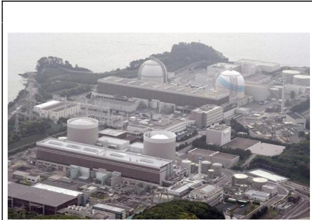
Genkai Plant’s 4 Reactors are Close Together
