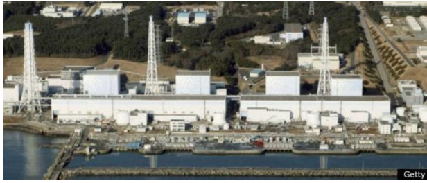
Fukushima Daiichi Nuclear Power Plant (before)
