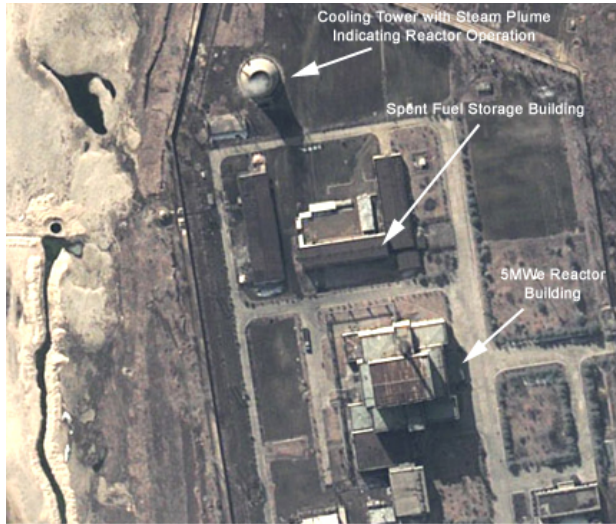
5 MWE REACTOR COMPLEX AT YONGBYON, DPRK
