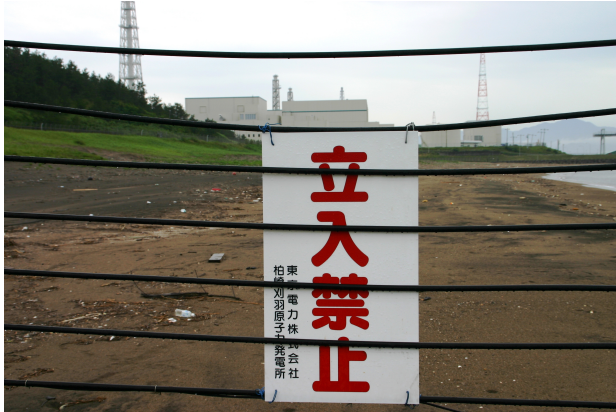
Kashiwazaki-Kariwa Nuclear Power Plant entrance days after the earthquake
