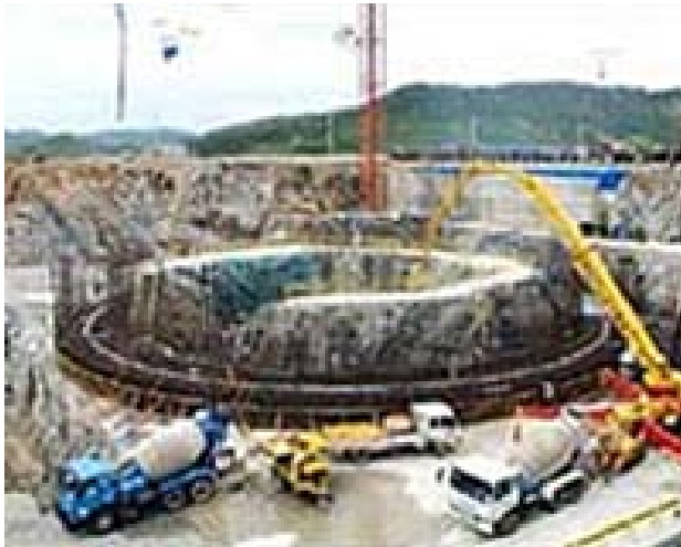
Incomplete light water reactor in North Korea
