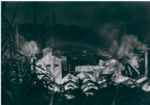
The Chisso Minamata plant
