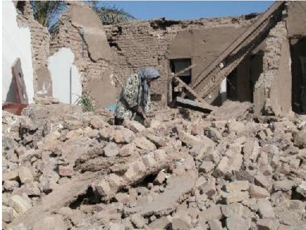
Bam Earthquake on Dec. 26, 2003.
