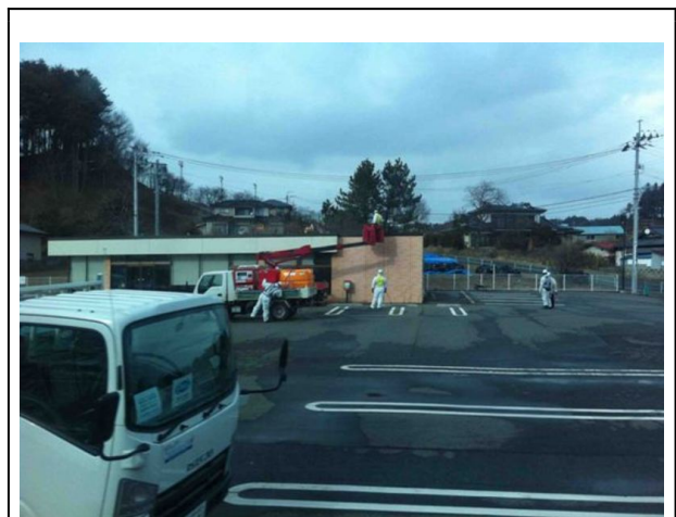
Decontamination work ( josen ) in Iidatemura, 13 January, 2012. (Photo: Kristopher Stevens)
