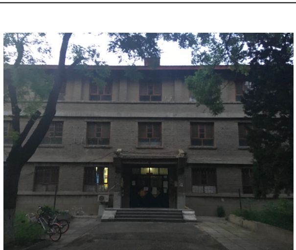
Old dorm slated for demolition
