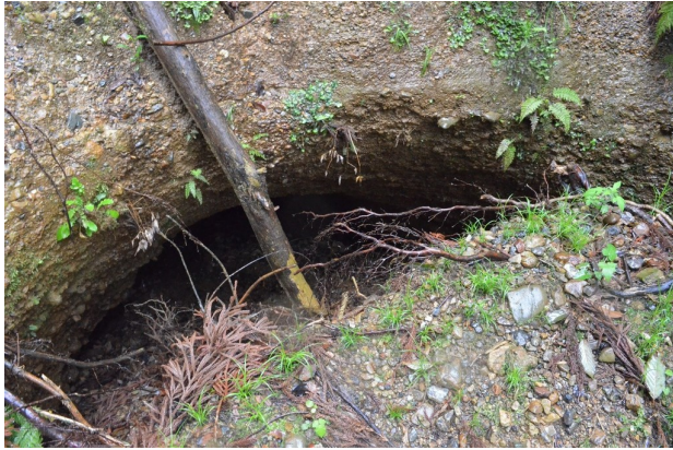
Photo 2: One of the Remaining Few Tunnel Entrances of the Tachisō
