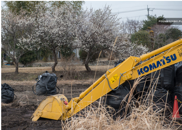
Landfill bags with contaminated soil in Tomioka Decontamination of personal possessions
