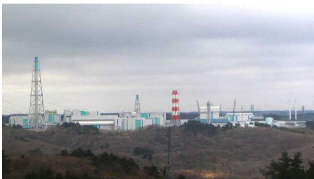
Ikata nuclear power plant (Shikoku): reactor 1 to be decommissioned, center bottom
