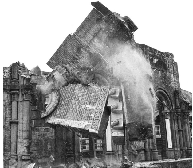
Dismantling of Remnants of the Cathedral Photo courtesy of Itaru Takahara
