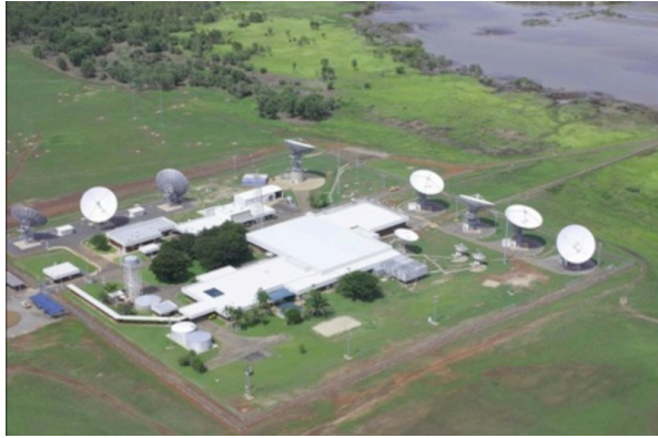
Shoal Bay Receiving Station, January 2013
