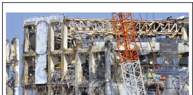
Reactor # 4 at Fukushima Daiichi
