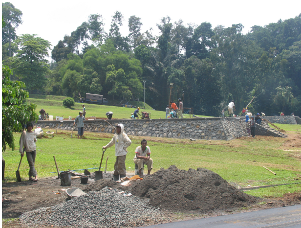
Construction at the Bogor Botanical Garden
