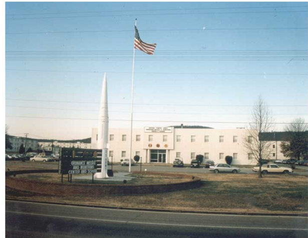
Headquarters Building, Redstone Arsenal, Huntsville, Alabama U.S. Army Aviation and Missile Command photo
