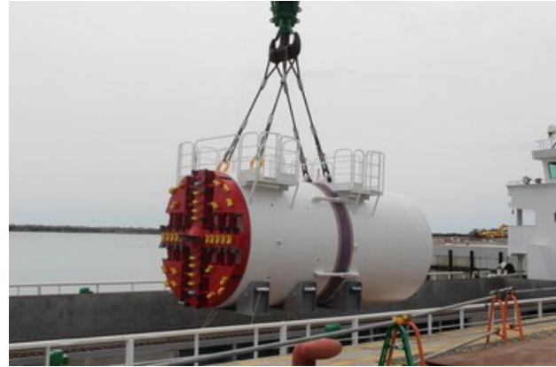
Water discharge system under construction. April 2022. Credit:TEPCO
