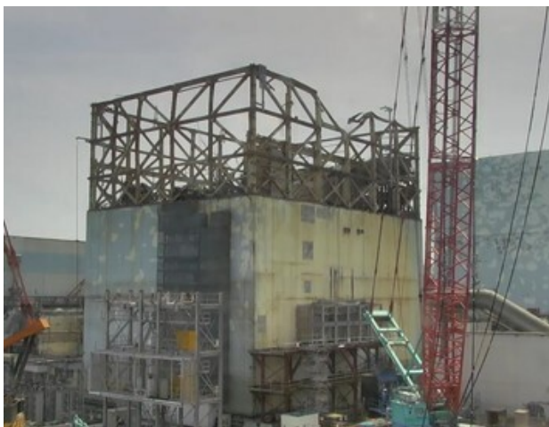
Reactor 1 before cover installed in October 2011. Credit: TEPCO
