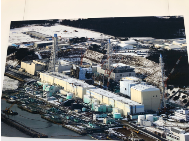
Undated photo of 4 reactors, here with Reactor 1 (at right) covered. The cover was installed in October 2011 but the roof was removed in 2015, while the wall panels were removed in 2021 in preparation for installing a new building cover in 2023 to facilitate spent fuel rod removal. The other three reactors are now all shrouded (see below). Credit: The Great East Japan Earthquake and Nuclear Disaster Museum.
