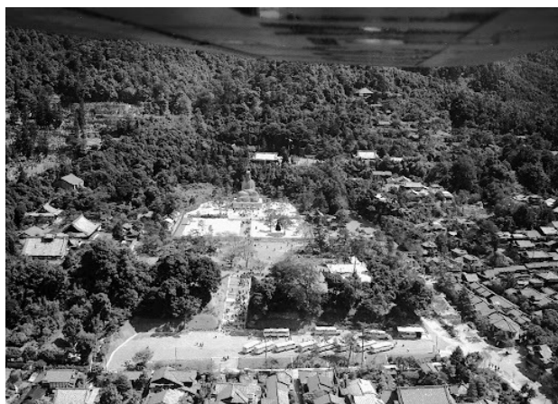
Figure 2: Ryōzen Kannon and surroundings on 29 September 1956 (Yomiuri Shashinkan). The statue is in the middle, surrounded by buildings of Kōdai-
