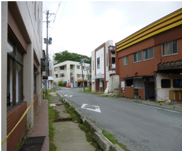
Fig. 6 Tomioka in June 2013: due to the high contamination background radiation, there is no one in town, but buildings of the central street still remains. (Photo: Paul Jobin)
