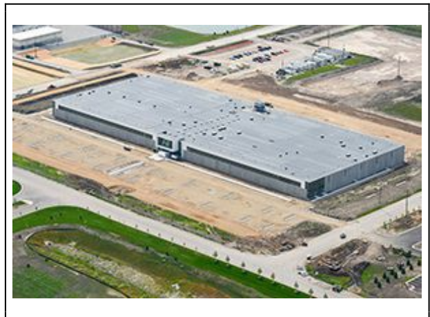
Smart manufacturing center: A 260,000-square-foot facility built by Fii, which says it will use it to manufacture server parts and employ 300 to 500
