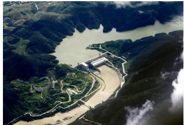
Jinghong hydropower station on the Lancang River in China (Image: Alamy)
