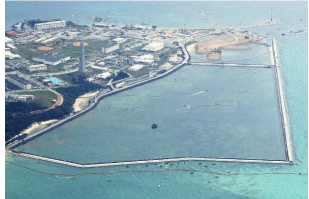
Henoko base construction
