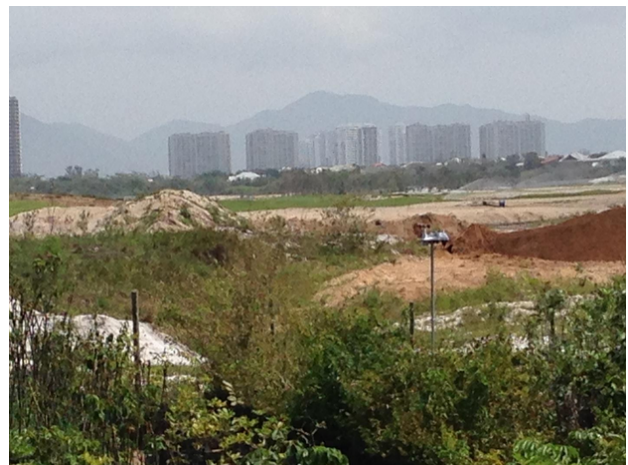
Olympic Golf course under construction
