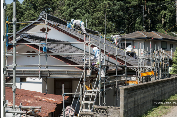
The roofs of all the buildings are hand-cleaned tile by tile.
