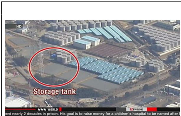
Leaking storage tank and TEPCO attempts to contain contaminated water at Fukushima Daiichi (NHK)
