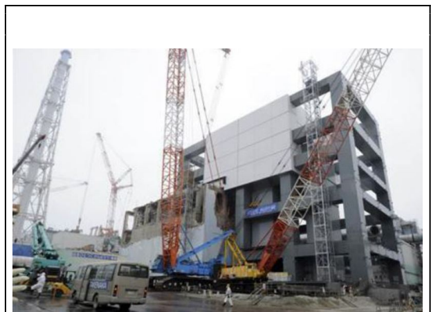
Tepeco preparing to remove irradiated fuel
