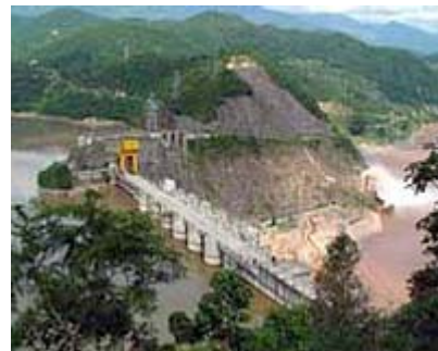
The Manwan Dam
