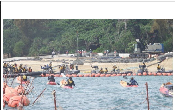
Construction begins as protestors kayaks cry out “stop!” April 25, 2017 ©Tsuyoshi Kitaueda
