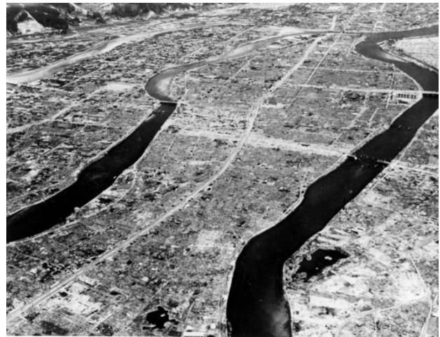
Aerial view of Hiroshima after the bombing.
