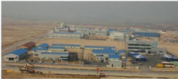
<Gaeseong Industrial Complex>
