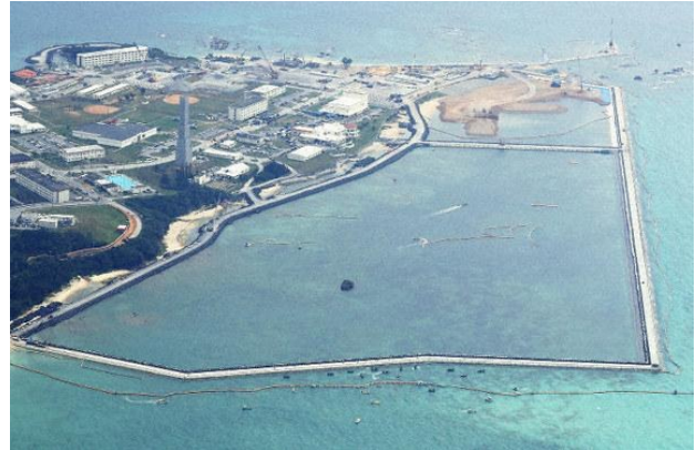
Henoko base construction
