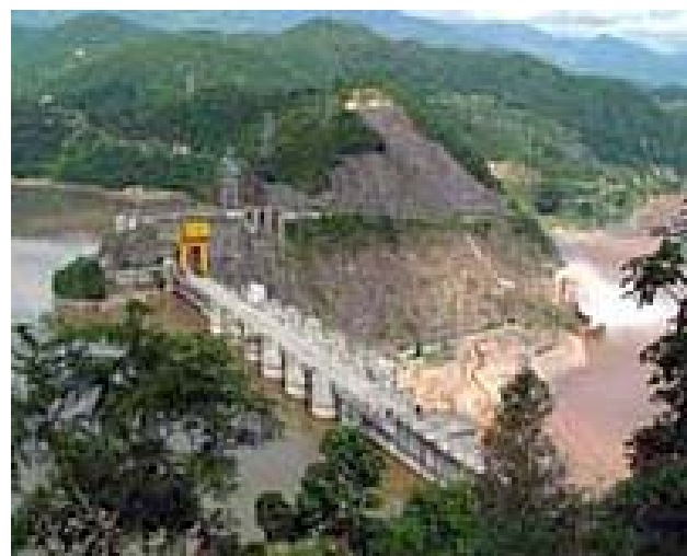
The Manwan Dam
