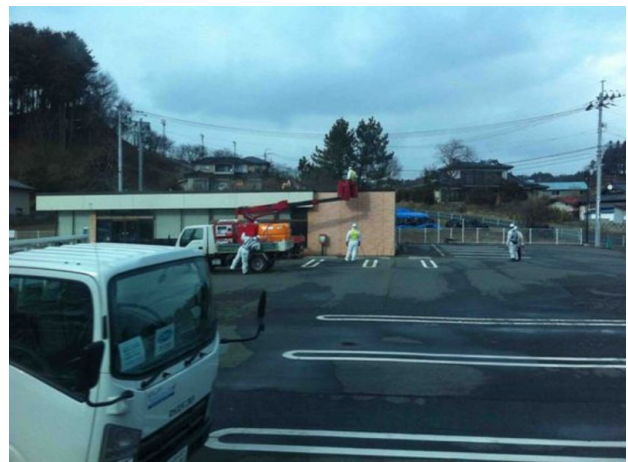
Decontamination work ( josen ) in Iidatemura, 13 January, 2012. (Photo: Kristopher Stevens)
